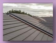
**Roof -** The roof is the most vulnerable part of your home. Homes with wood or shingle roofs are at high risk of being destroyed during a wildfire. Build your roof or re-roof with materials such as composition, metal or tile. Block any spaces between roof decking and covering to prevent embers from catching.
