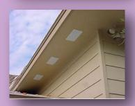
**Walls -** Wood products, such as boards, panels or shingles, are common siding materials. However, they are flammable and not good choices for fire-prone areas. Build or remodel your walls with ignition resistant building materials, such as stucco, fiber cement wall siding, fire retardant, treated wood, or other approved materials. Be sure to extend materials from the foundation to the roof.
