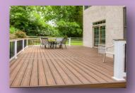
**Decks -** Surfaces within 10 feet of the building should be built with ignition-resistant, non-combustible or other approved materials. Ensure that all combustible items are removed from underneath your deck.
